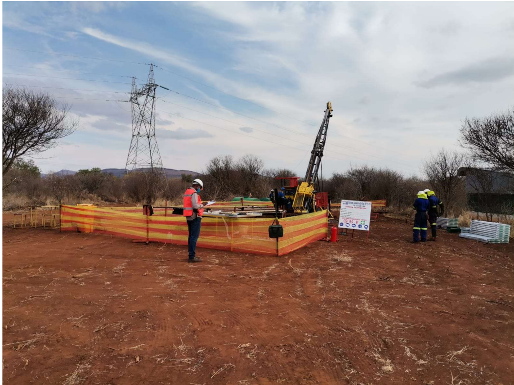
Figure 1: Drill rig site establishment at the Zeb Project.
